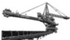
Stacker and Reclaimer
